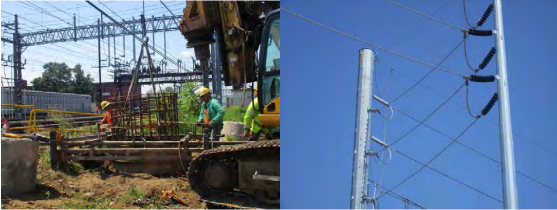
Setting rebar cage at 815N and bypass at Baird Substation
