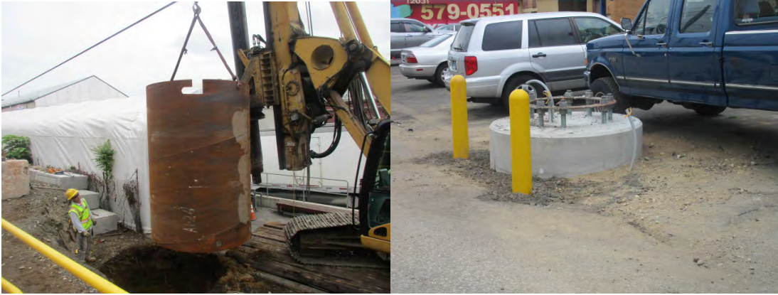
Setting caisson at 826S and bollards at 793N
