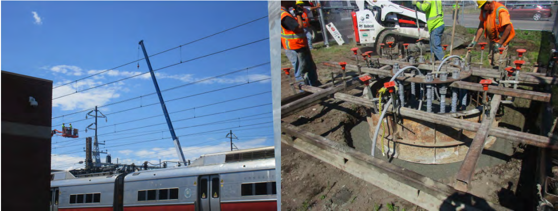
Bonnet removals in rail yard and pouring concrete for 801N
