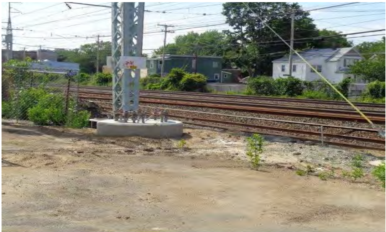
Foundation for Structure 820S
