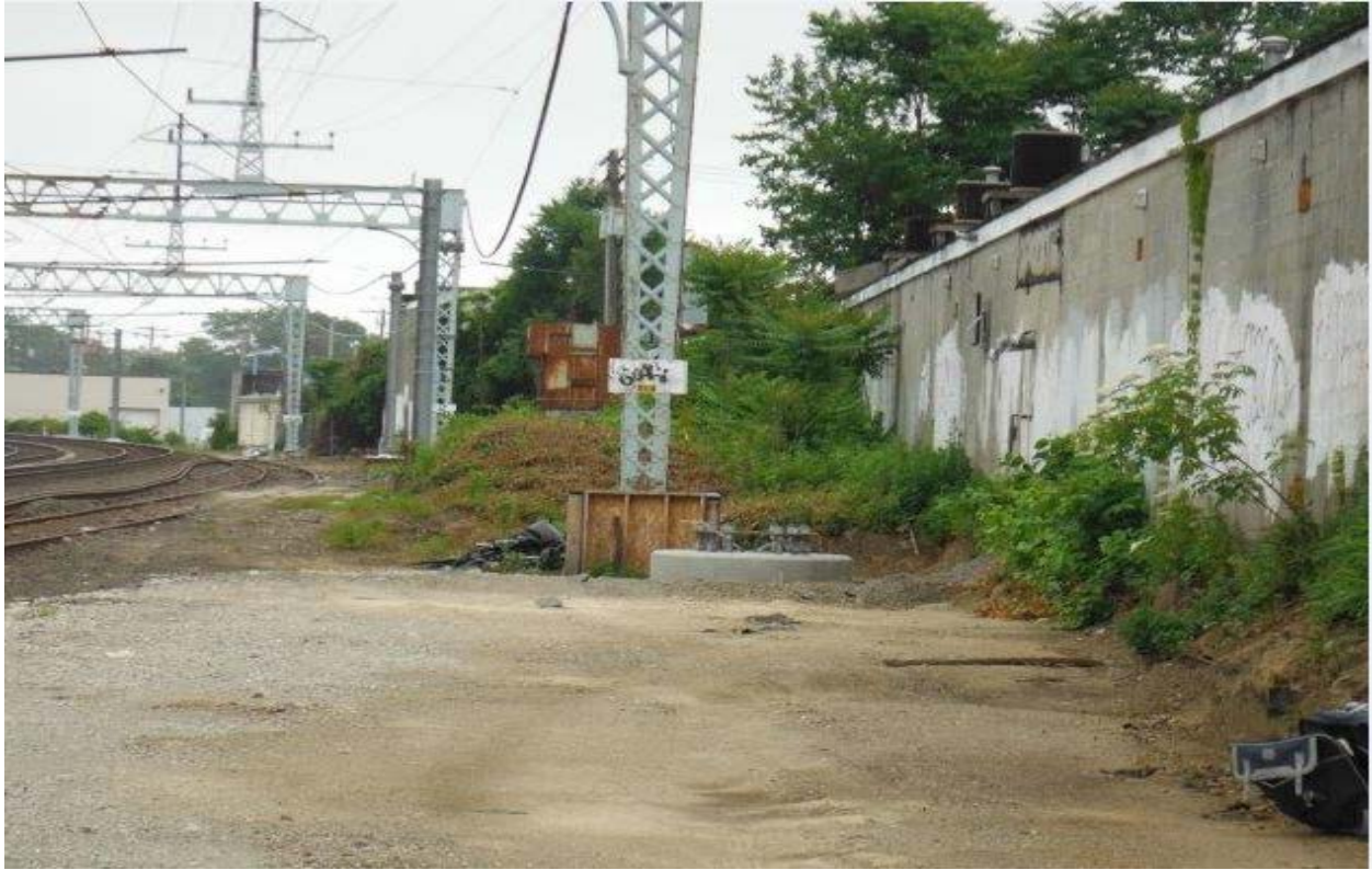
Foundation for Structure 817S
