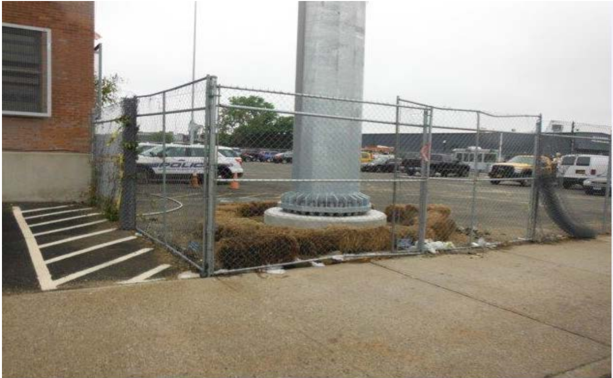
Structure 806S with erosion and sediment controls
