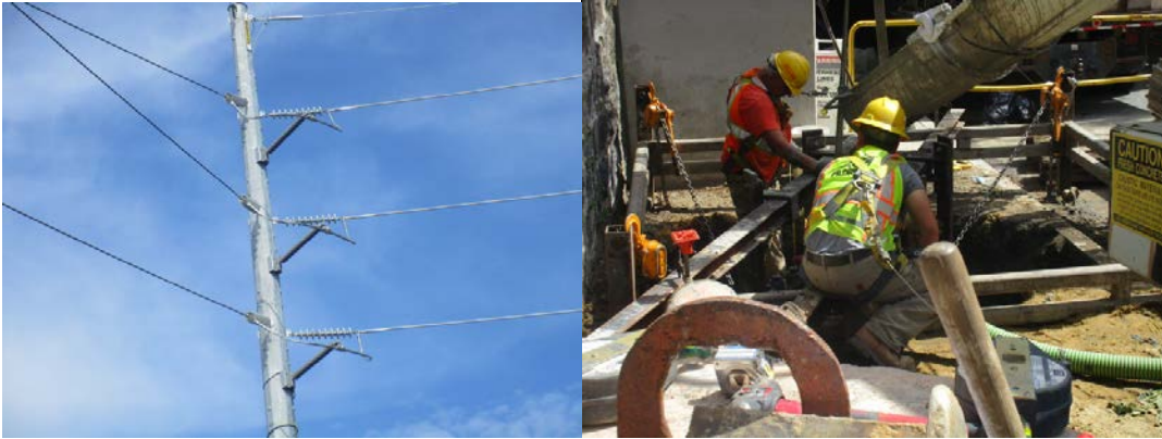
Dead ends and jumpers installed at 805S and pouring concrete for 789N
