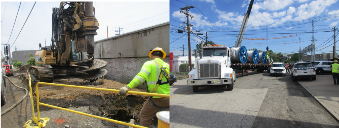
Drilling foundation 822S and stringing setup at structure 806S
