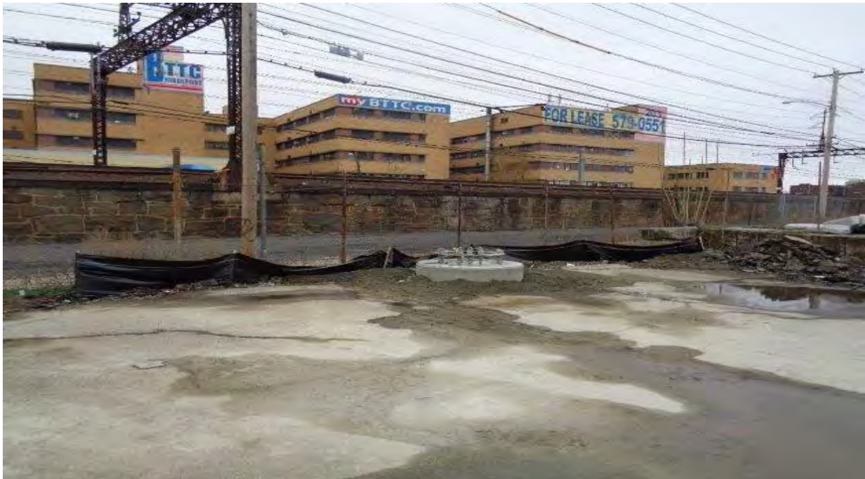
Foundation for Structure 793S
