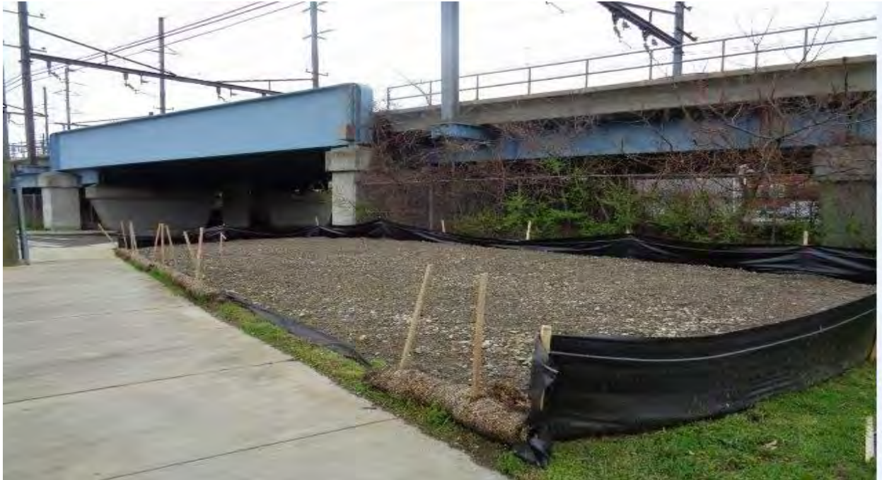
Work pad for Structure 785N
