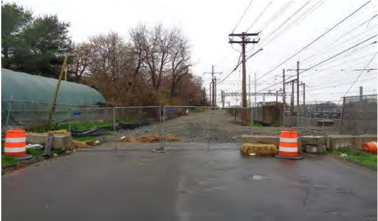
Access road for Structure(s) 824N and 825N
