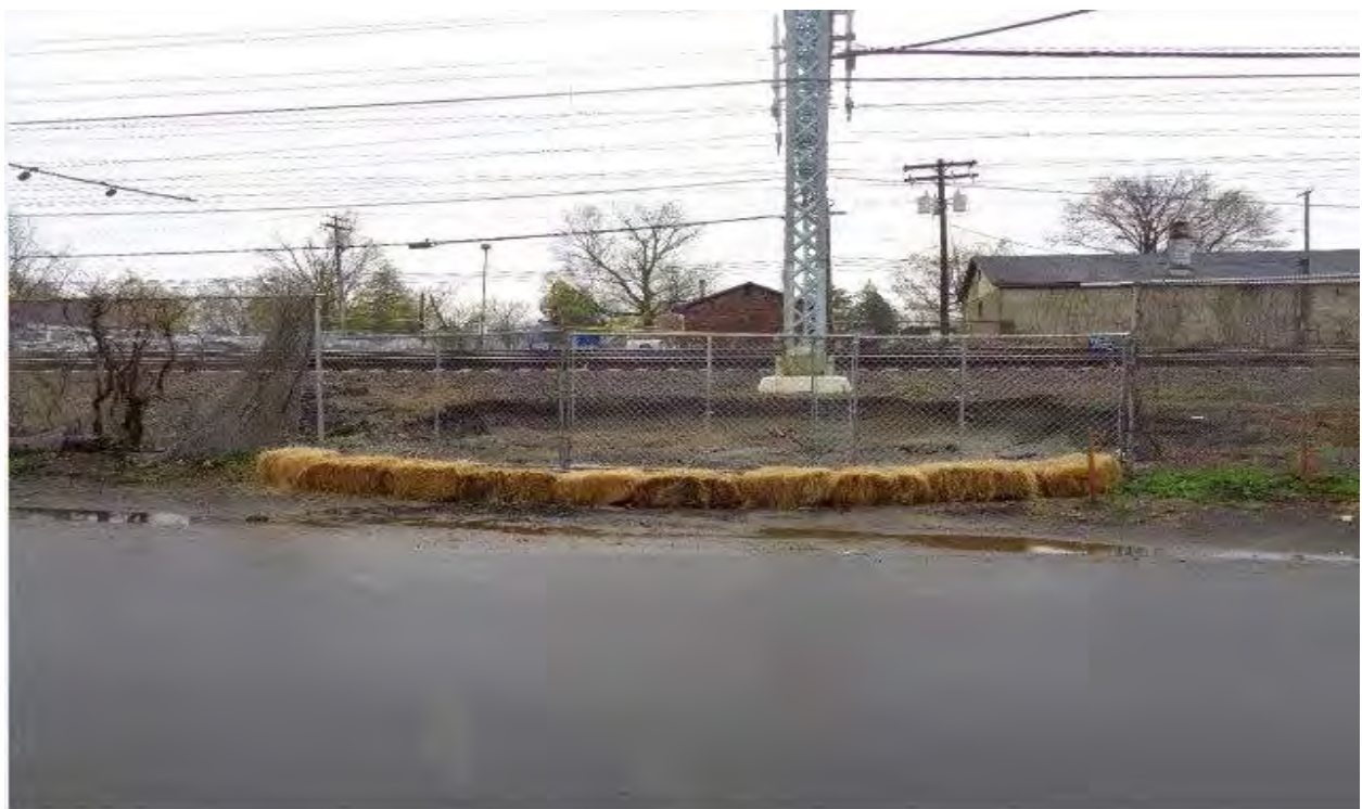
Work pad for Structure 819N
