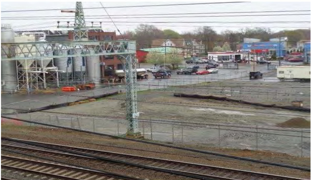
Work area for Structure(s) 824S and 825S
