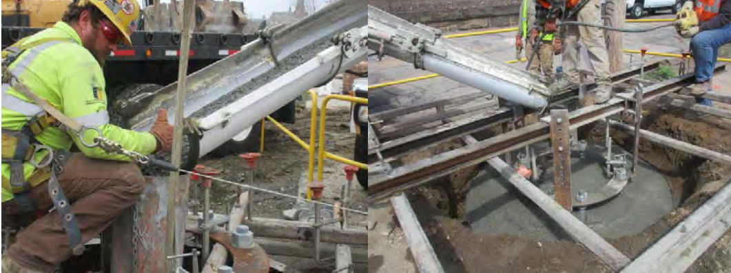
Pouring foundations 799S and 798S
