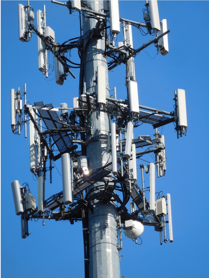
Photo 1: Photo illustrating the Monopole with Appurtenances shown.
