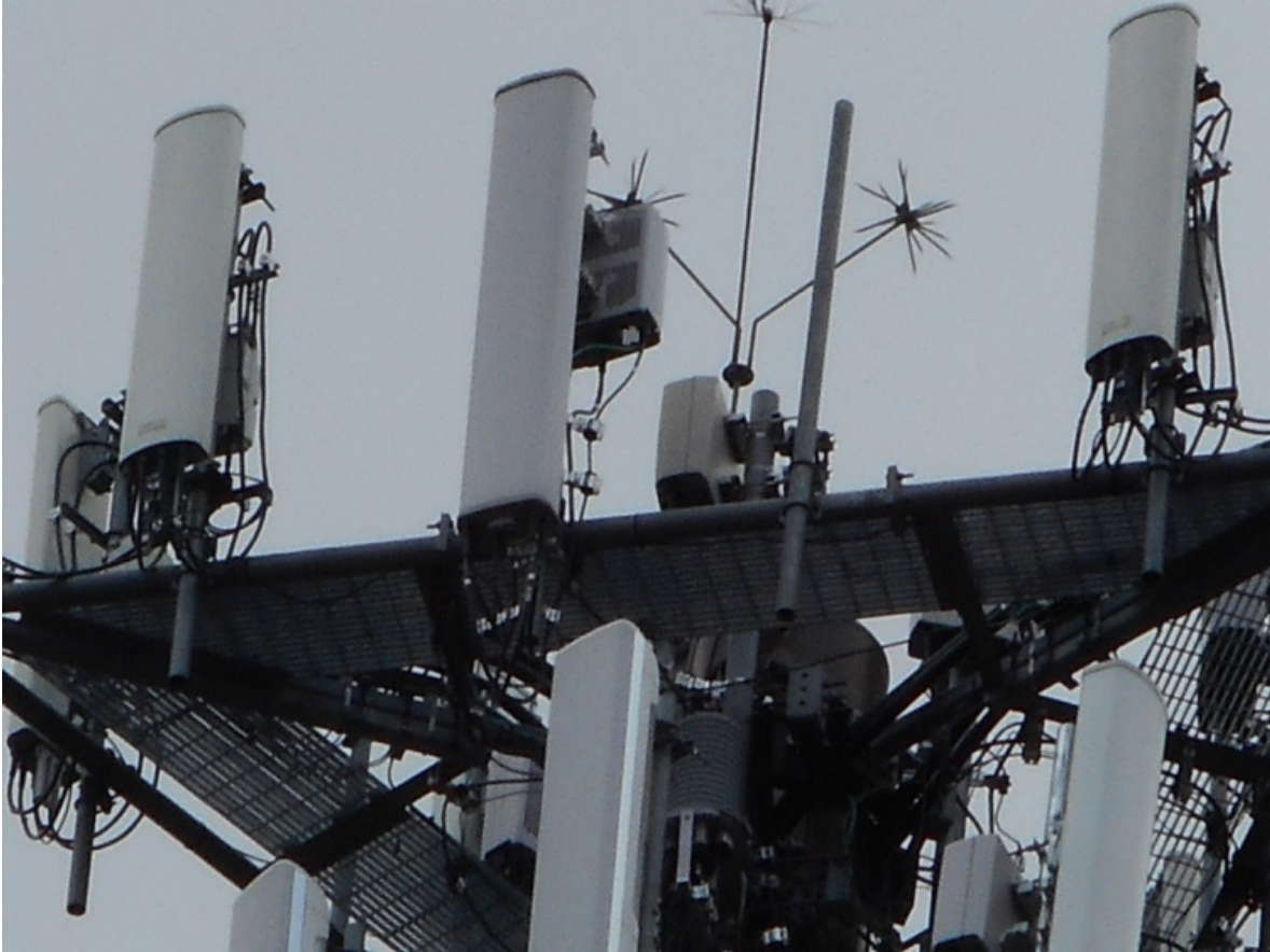
Photo 1: Photo illustrating the monopole with Appurtenances shown.
