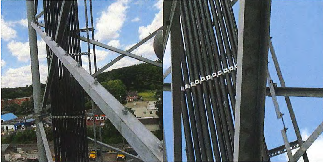
All Added Diagonals Installed Correctly
