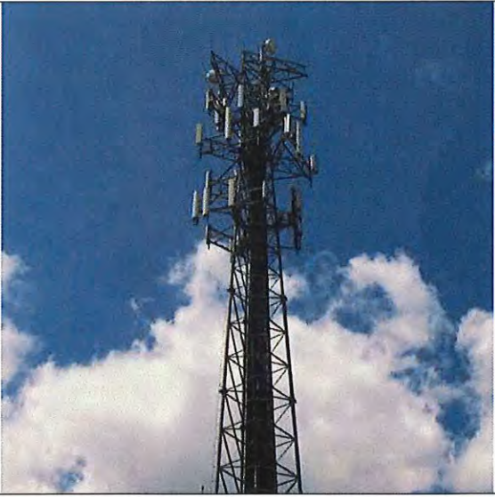
Top Half of Tower
