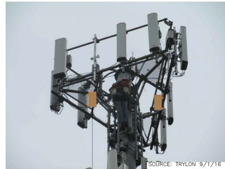
PROPOSED LTE RRUS-32 B2 & RRUS-32 LOCATED ON NEW RRU BRACKET, BACK-TO-BACK (TYP. 2 PER SECTOR, 6 TOTAL)
