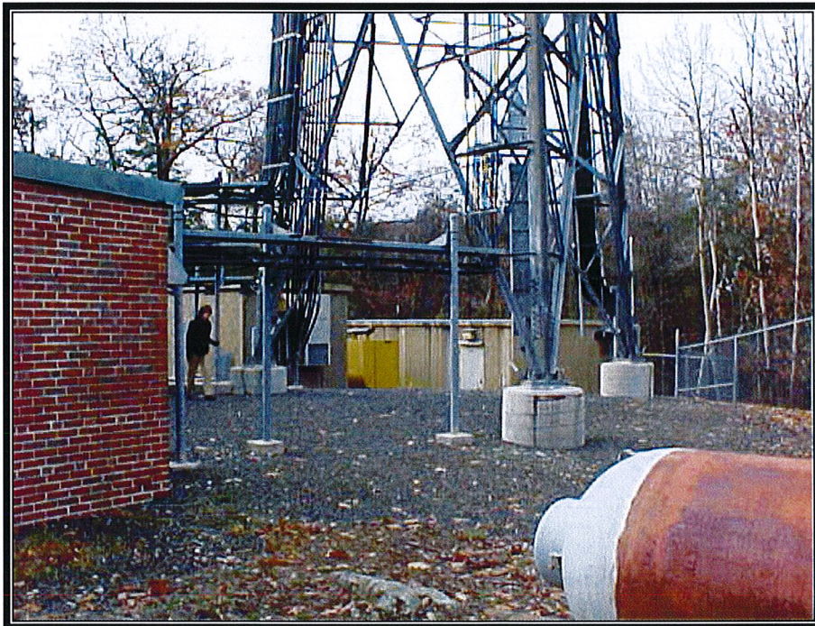
Photo 2-2. View of the Tower Base
