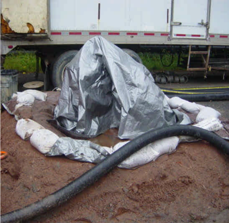
Secondary containment has been provided for two 55-gallon drums located in the staging area on the east side of the river
