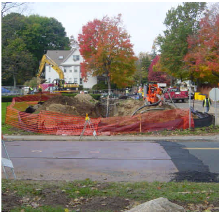
On the west side of the Saugatuck river, Lincoln St. has been closed as conduit sections are being staged and fused together as crews prepare for the conduit pull. The drilling/recycling pit has been expanded as additional soil continues to slough into the pit. Steel plates have been proactively installed along Riverside Avenue to distribute vehicle loads over the boring.
