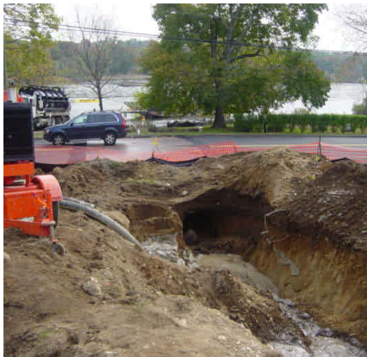
On the west side of the Saugatuck river, Lincoln St. has been closed as conduit sections are being staged and fused together as crews prepare for the conduit pull. The drilling/recycling pit has been expanded as additional soil continues to slough into the pit. Steel plates have been proactively installed along Riverside Avenue to distribute vehicle loads over the boring.
