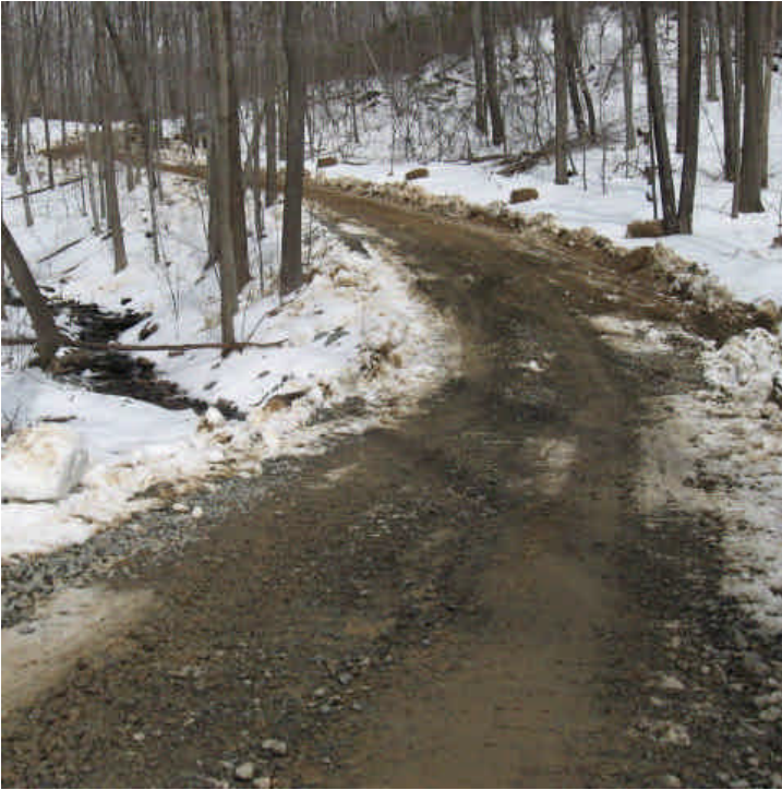
Cow Path Lane: View of the access road at the stream crossing on 3/19/07
