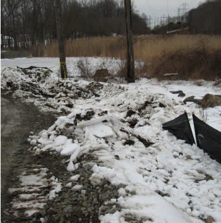
Whealers Farm Road (Milford): Snow was plowed over the silt fence off Wheelers Farm (west) on 3/19/07
