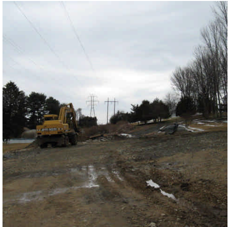
Hunting Hill Place (Orange): Foundation drilling/pouring appears to be complete. 3/23/07
