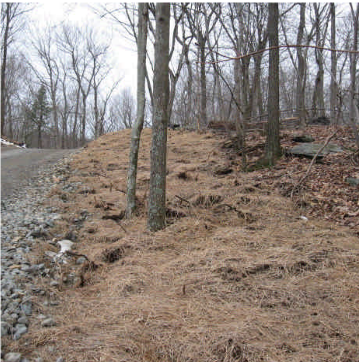
Cow Path Lane: Mulch was applied to the side slopes of the access road near the stream crossing 3/23/07.
