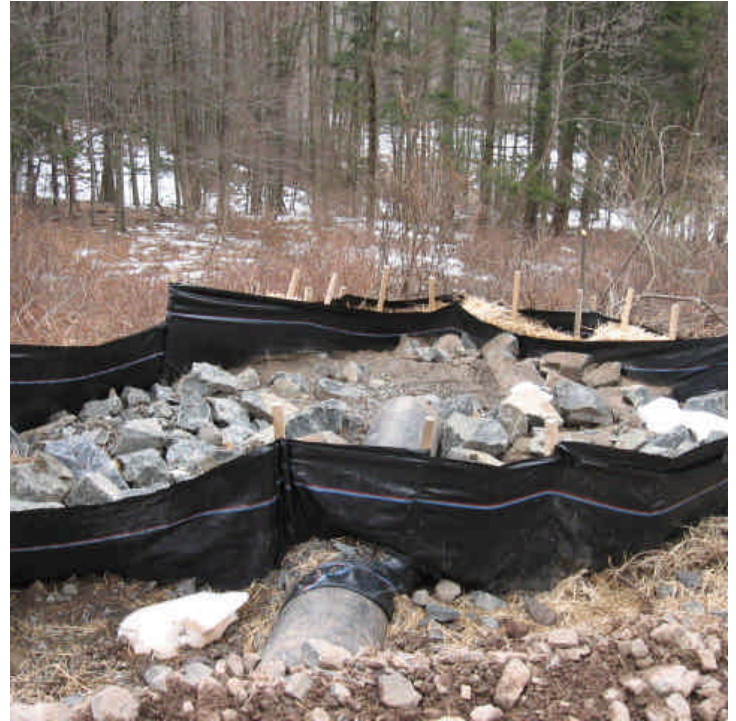
SCRWA, Morris to Dillon St: Erosion controls remain intact along the access roads, culvert location, and throughout the ROW. Sediment has built up in the stone trap at the culvert outlet. 3/23/07.
