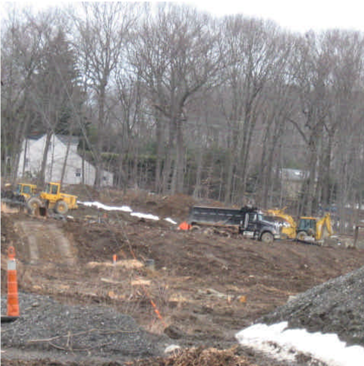
Work associated with the relocation of Shelland Street continues. 3/23/07.
