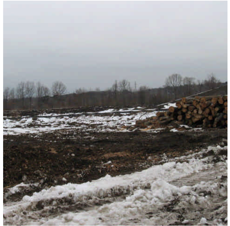
View of the clearing at the East Devon Substation site. 3/19/07.
