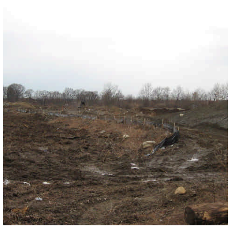
View of the ongoing clearing and grading activities. 3/23/07.
