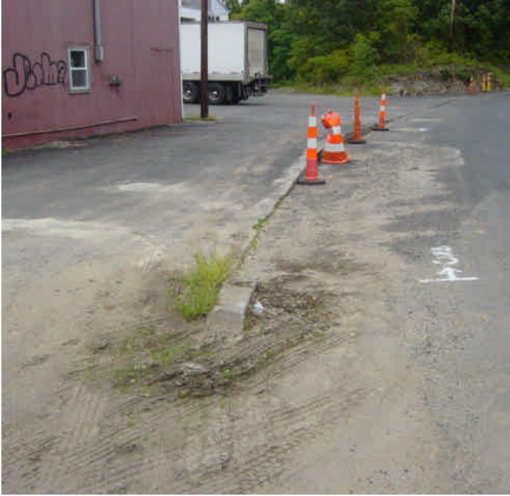
Sediment was observed along the curb line near the Metro North HDD staging area off of Naugatuck Ave. This material may not be project related.
