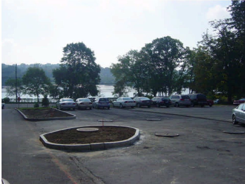
On the west side of the Saugatuck River, stone curbing has been reset and the parking lot received a base coat of pavement.
