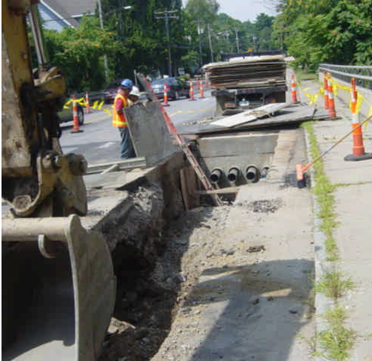
Tie-in work was occurring at the Mill River (Southport Harbor) Bridge Attachment. Work did not appear to impact the River. A filter barrier is in place in the channel.
