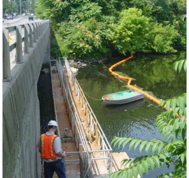
Tie-in work was occurring at the Mill River (Southport Harbor) Bridge Attachment. Work did not appear to impact the River. A filter barrier is in place in the channel.
