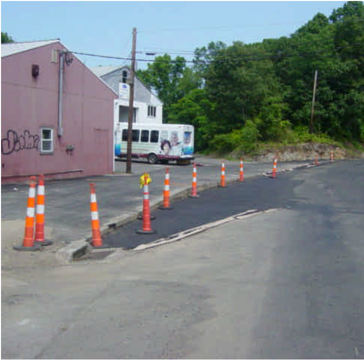
HDD work at the Metro North R.R. is complete. The circuits have been tied in on the north side. The roadway has been paved. A small area was re-graded to promote drainage. Accumulated sediment appears to have been swept near the end of the driveway adjacent to the catch basin.
