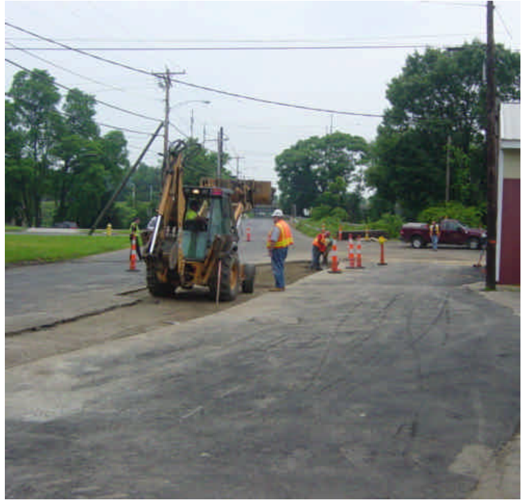
HDD work at the Metro North R.R. is complete. The circuits have been tied in on the north side. The roadway has been partially paved except for a small area which was being regraded to ensure proper drainage. Sediment has accumulated near the end of the driveway adjacent to the catch basin which did not have controls in place.
