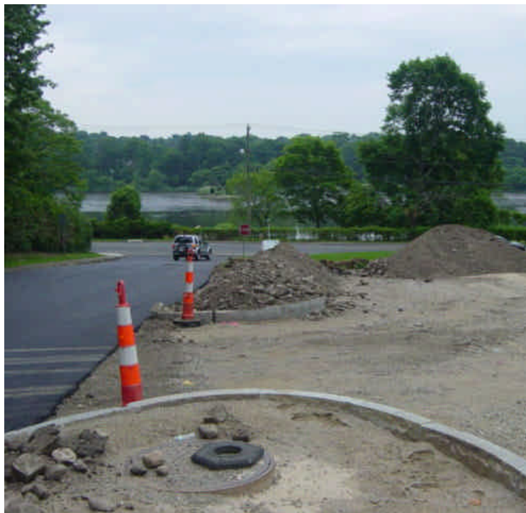
On the west side of the Saugatuck River, the portions of the work area that were restored are vegetated. The adjacent area is still waiting to be paved. Stone curbing has been set and soil has been stockpiled in these areas. Minor tracking was observed on Lincoln St. Accumulated sediment at the intersection of Lincoln St. and Riverside Ave. has been swept. This area has been scheduled for pavement for several months.
