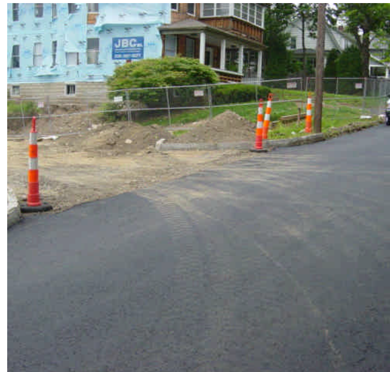
On the west side of the Saugatuck River, the portions of the work area that were restored are vegetated. The adjacent area is still waiting to be paved. Stone curbing has been set and soil has been stockpiled in these areas. Minor tracking was observed on Lincoln St. Accumulated sediment at the intersection of Lincoln St. and Riverside Ave. has been swept. This area has been scheduled for pavement for several months.
