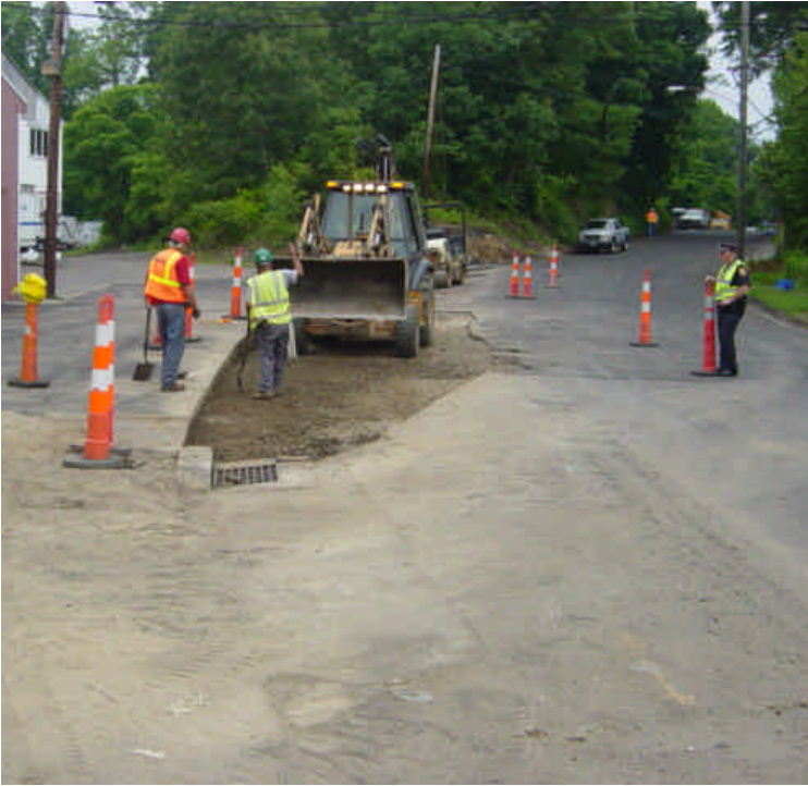
HDD work at the Metro North R.R. is complete. The circuits have been tied in on the north side. The roadway has been partially paved except for a small area which was being regraded to ensure proper drainage. Sediment has accumulated near the end of the driveway adjacent to the catch basin which did not have controls in place.
