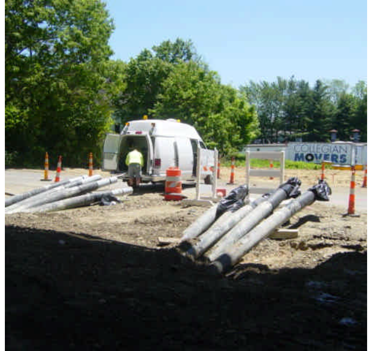
Metro North RR: Conduit has been pulled through the second boring and the drill pits have been partially backfilled. Electrical contractors were on site proofing the lines. The catch basin on the north side remains unprotected.
