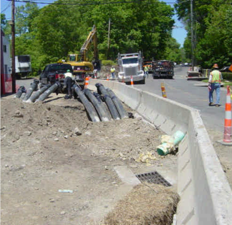
Metro North RR: Conduit has been pulled through the second boring and the drill pits have been partially backfilled. Electrical contractors were on site proofing the lines. The catch basin on the north side remains unprotected.
