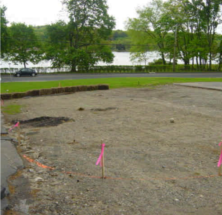
Staging area on the west side of the Saugatuck River has been partially restored. The area has been staked out in preparation for paving. Paving has been scheduled for a number of weeks but has not yet occurred.
