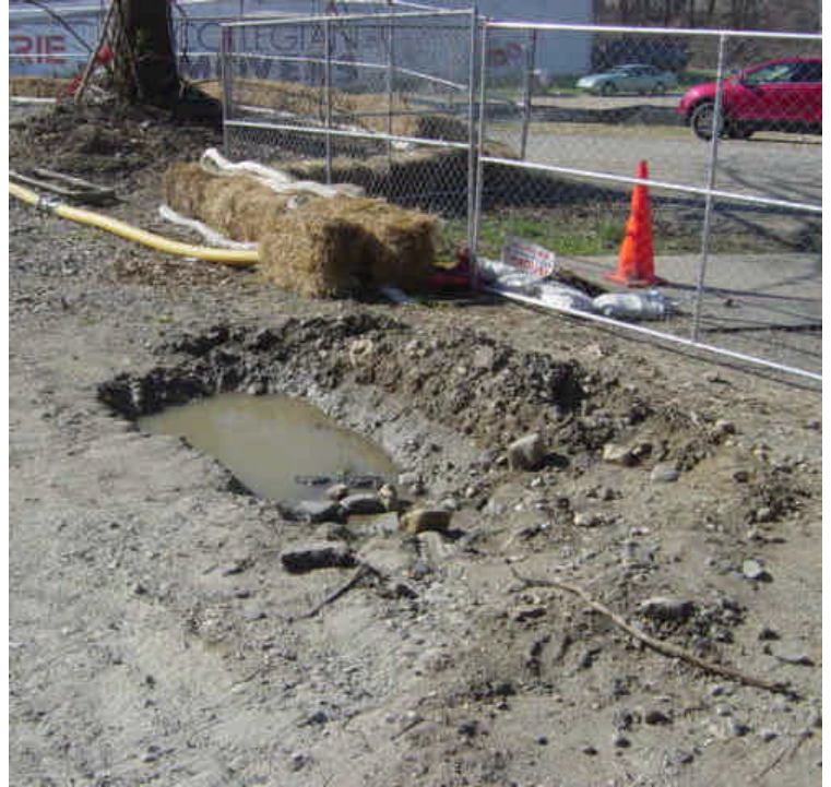
Conduit has been pulled through the first of two borings at the Metro North Railroad Crossing in Milford and there was no activity at the time of the inspection. A minor amount of slurry material was observed along the curb line along Nauagtick Ave. and the adjacent catch basin was not protected. A small pit has been excavated in the staging area but the material appears to be adequately contained at this time.
