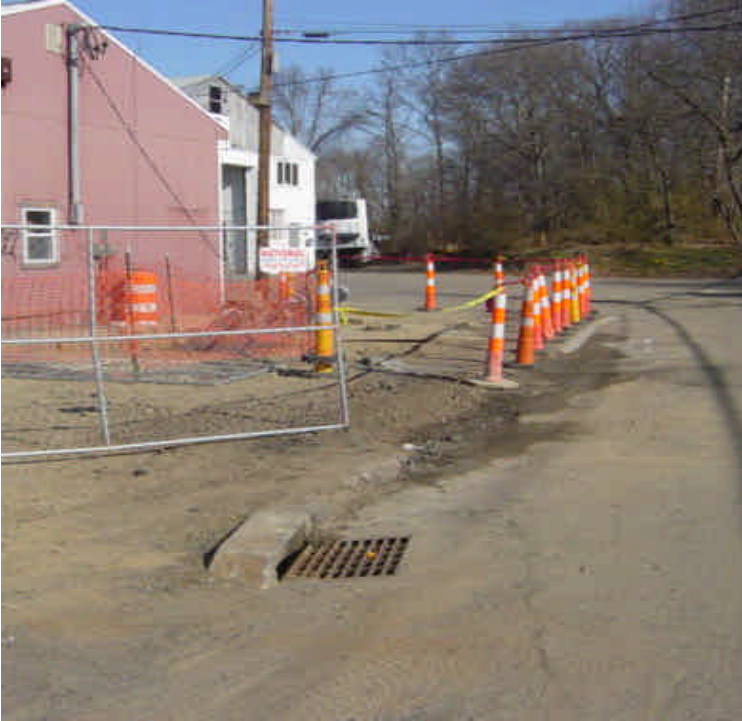
Conduit has been pulled through the first of two borings at the Metro North Railroad Crossing in Milford and there was no activity at the time of the inspection. A minor amount of slurry material was observed along the curb line along Nauagtick Ave. and the adjacent catch basin was not protected. A small pit has been excavated in the staging area but the material appears to be adequately contained at this time.
