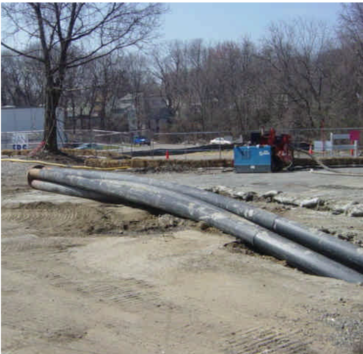
Conduit has been pulled through the first of two borings at the Metro North Railroad Crossing in Milford. A minor amount of slurry material was observed near the perimeter of the staging area, but it was being adequately contained by a haybale barrier.
