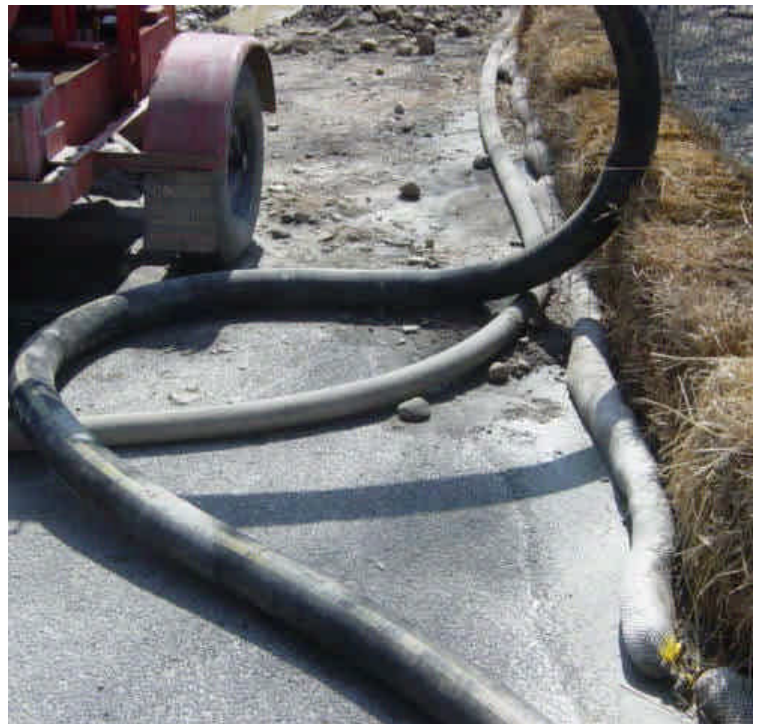
Conduit has been pulled through the first of two borings at the Metro North Railroad Crossing in Milford. A minor amount of slurry material was observed near the perimeter of the staging area, but it was being adequately contained by a haybale barrier.
