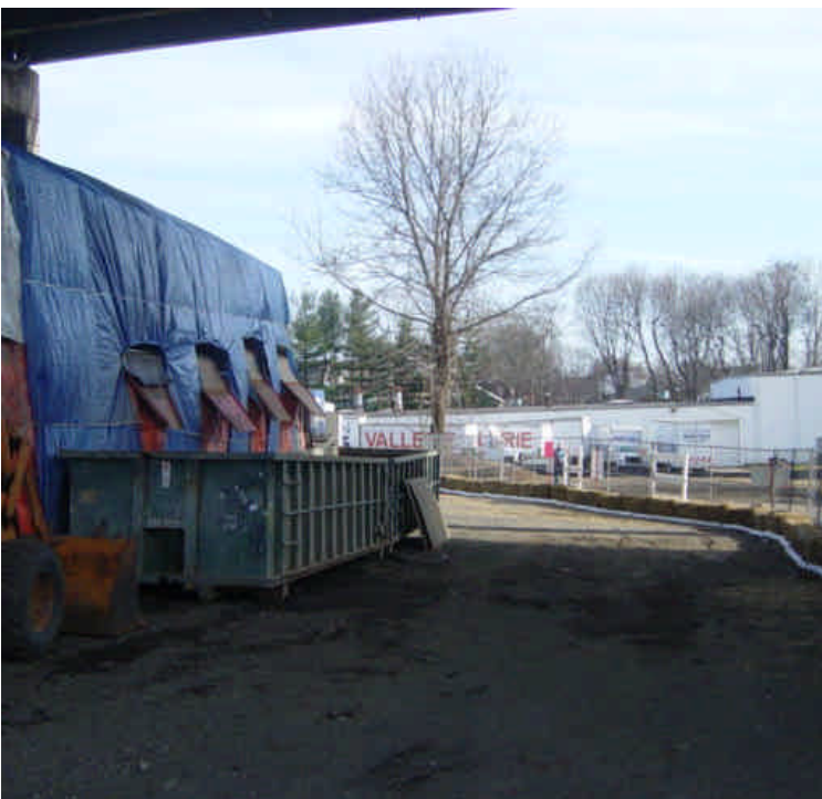
A staging area has been set-up on the south side of the Metro North R.R. in Milford. The staging area has been surrounded by haybales and a filter boom. A temporary access drive has been cut to provide access to the boat launch area. Drilling equipment is being set-up including a bentonite reclamation machine under the I-95 overpass.
