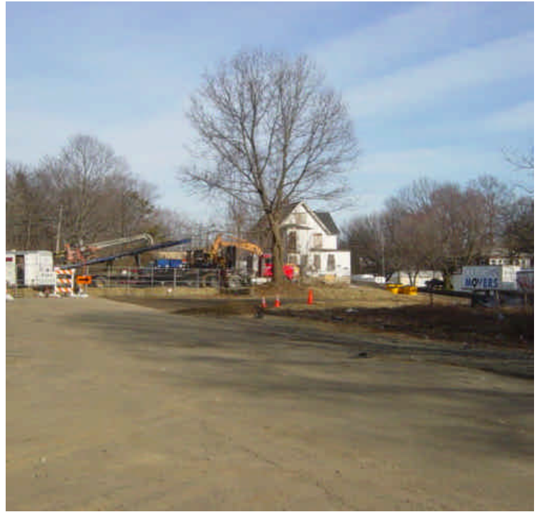
A staging area has been set-up on the south side of the Metro North R.R. in Milford. The staging area has been surrounded by haybales and a filter boom. A temporary access drive has been cut to provide access to the boat launch area. Drilling equipment is being set-up including a bentonite reclamation machine under the I-95 overpass.
