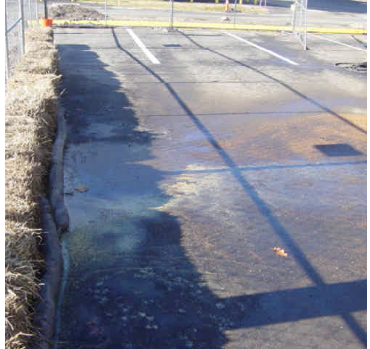
The spill/leak that has been observed for the last two weeks near the generator trailer is worsening. Absorbent material remains spread over some portions of the spill and absorbent booms were in use. However, material continues to leak and a small pool of yellow liquid was observed adjacent to the hay bale barrier. Repair the leaking machinery ASAP and provide additional containment and clean-up.
