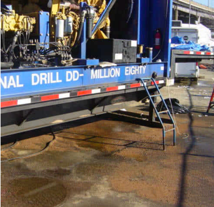
The spill/leak that has been observed for the last two weeks near the generator trailer is worsening. Absorbent material remains spread over some portions of the spill and absorbent booms were in use. However, material continues to leak and a small pool of yellow liquid was observed adjacent to the hay bale barrier. Repair the leaking machinery ASAP and provide additional containment and clean-up.
