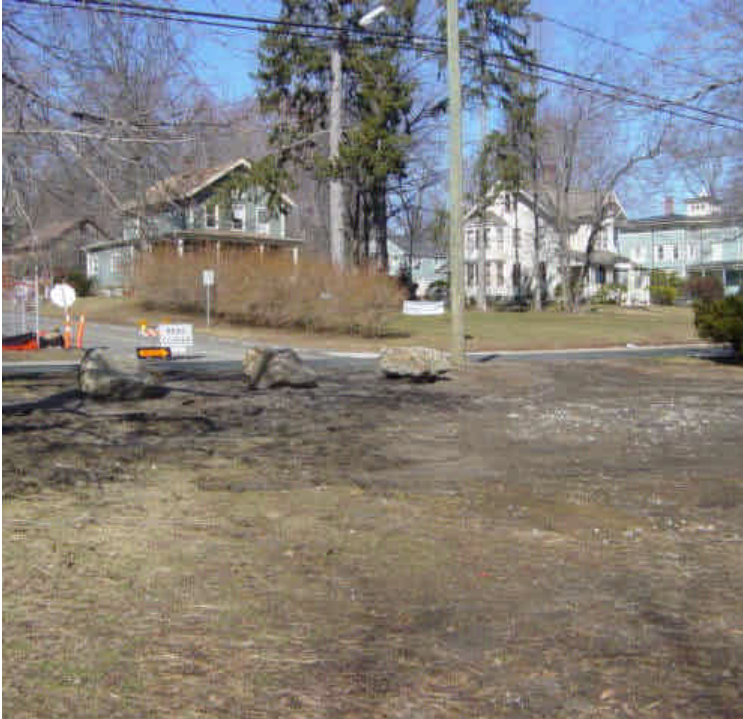
Clean-up efforts within the Saugatuck River have been completed. The crushed stone has been removed from the park area near Riverside Ave. where vacuum trucks had accessed the river. Minor ruts remains in this area. Final restoration will be needed during the growing season.
