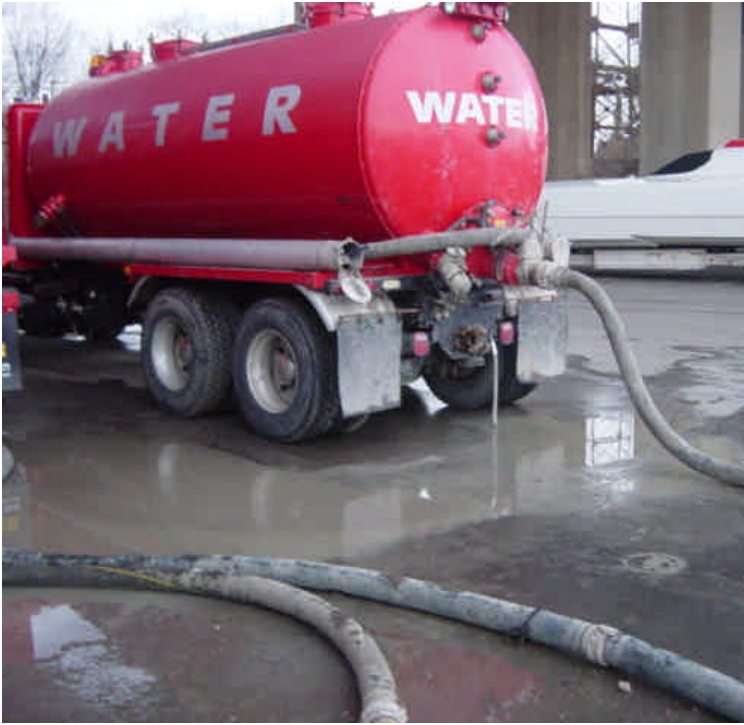
On the west side of the Housatonic River, a minor amount of incidental water/slurry was observed on the paved surface near the northeast corner of the staging area.
