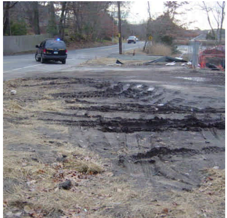
On the east side of the Saugatuck River, the drilling work has been completed and all of the equipment has been removed from the site. Heavy ruts were observed along the shoulder of Imperial Ave. (photo on the right). Chain link fencing was previously positioned in this area and had prevented vehicles from entering the staging area directly from Imperial Ave. The fence has since been relocated to around the drilling pits. (photo on the left).
