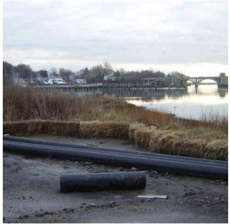
On the east side of the Housatonic River a haybale barrier remains in place near the end of the paved surface.
