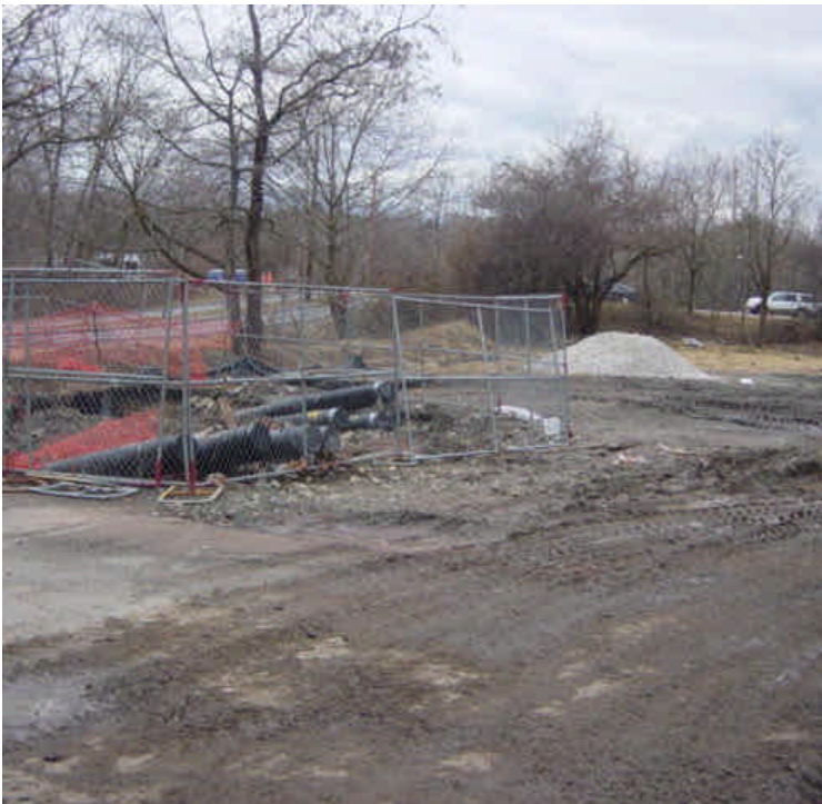
On the east side of the Saugatuck River, the drilling work has been completed and all of the equipment has been removed from the site. Heavy ruts were observed along the shoulder of Imperial Ave. (photo on the right). Chain link fencing was previously positioned in this area and had prevented vehicles from entering the staging area directly from Imperial Ave. The fence has since been relocated to around the drilling pits. (photo on the left).
