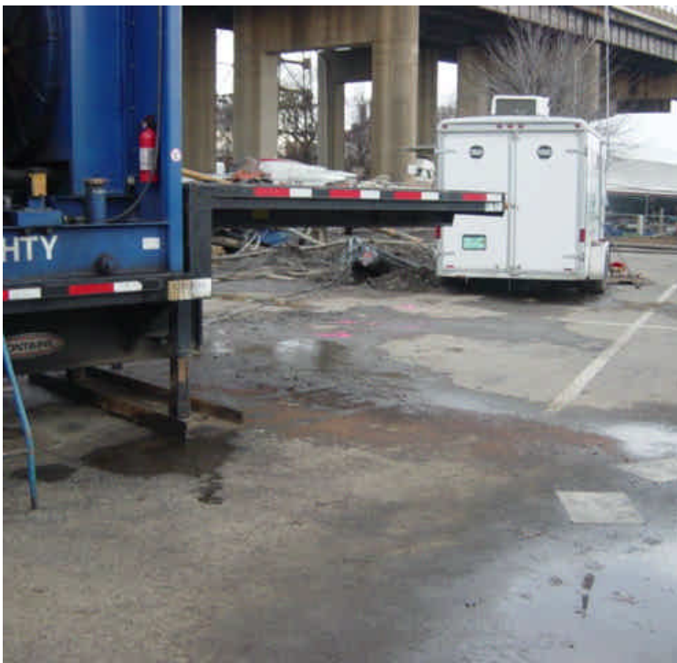
A spill/leak was observed near the generator trailer. Absorbent material appeared to be spread over most portions of the spill and absorbent booms were also utilized. Isolate the source of the spill/leak and provide containment and repair.
