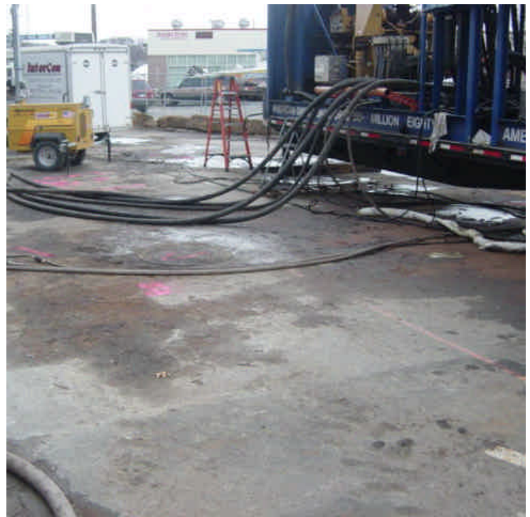
A spill/leak was observed near the generator trailer. Absorbent material appeared to be spread over most portions of the spill and absorbent booms were also utilized. Isolate the source of the spill/leak and provide containment and repair.
