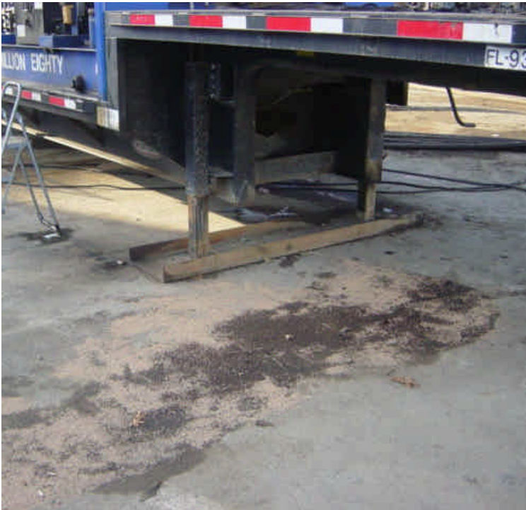
Spilled substance near the generator trailer appeared to be properly handled. At the time of the inspection, the spill was covered with an absorbent material.
