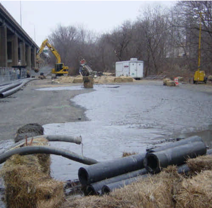
Drilling continues under the Housatonic River. Crews have been experiencing a loss of drilling fluid returns over the past several days, but divers have been surveying the area and there have been no signs of any frac-outs within the project limits. On the east side of the Housatonic River a large volume of drilling fluid was observed on the surface of the paved area. Hay bales were in place to contain the area and crews were working with vacuum trucks to remove the material.
