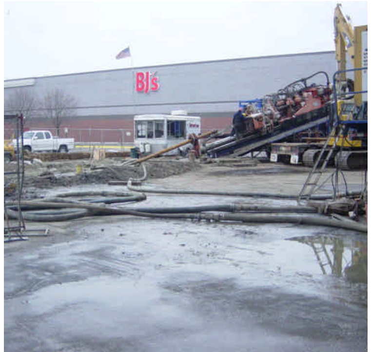
Drilling continues under the Housatonic River. Crews have been experiencing a loss of drilling fluid returns over the past several days, but divers have been surveying the area and there have been no signs of any frac-outs within the project limits. On the east side of the Housatonic River a large volume of drilling fluid was observed on the surface of the paved area. Hay bales were in place to contain the area and crews were working with vacuum trucks to remove the material.
