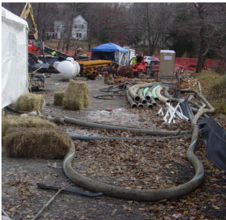
Slurry material was previously spilled in the staging area on the east side of the Saugatuck River near the bentonite reclamation machine, the drilling pit, and a frac tank.
