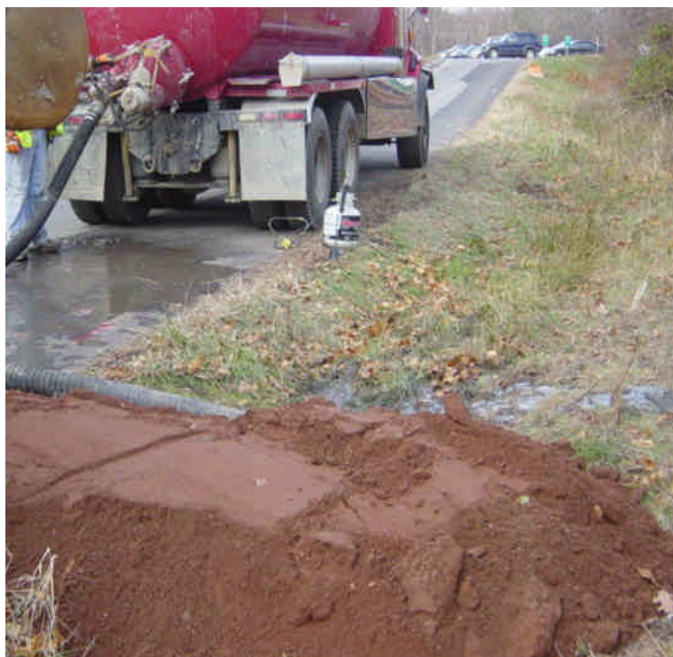
On the east side of the Saugatuck River, a small frac out occurred near the access driveway adjacent to the staging area. A sand berm was in place to contain the material and crews appeared to be adequately handling the situation. Ensure exposed sand from the berm will not migrate toward the river.
