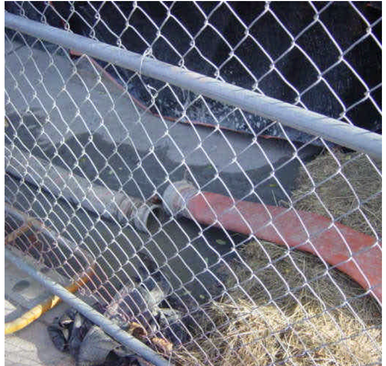
Hoses behind the betonite reclamation machine near Ash Creek have been disconnected, causing drilling material to spill onto the roadway. Although the adjacent catch basin is protected, attempt to sweep up the residue.
