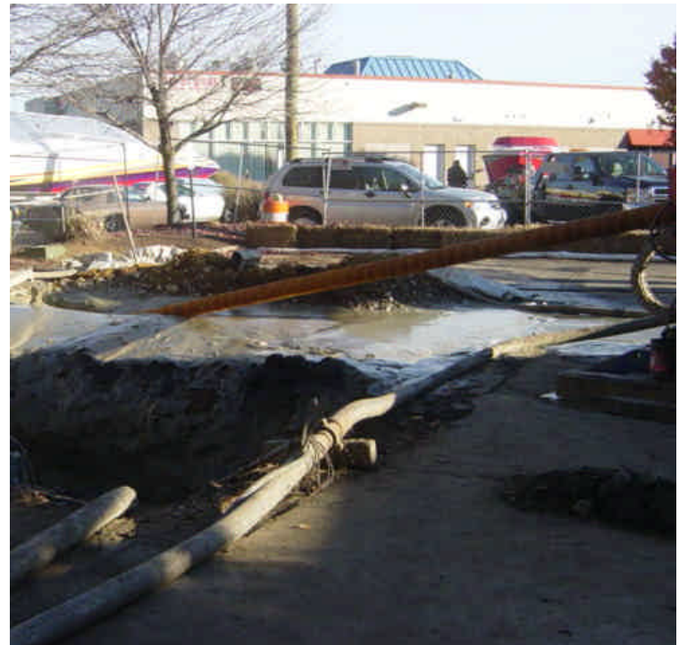
Hoses behind the betonite reclamation machine near Ash Creek have been disconnected, causing drilling material to spill onto the roadway. Although the adjacent catch basin is protected, attempt to sweep up the residue.
