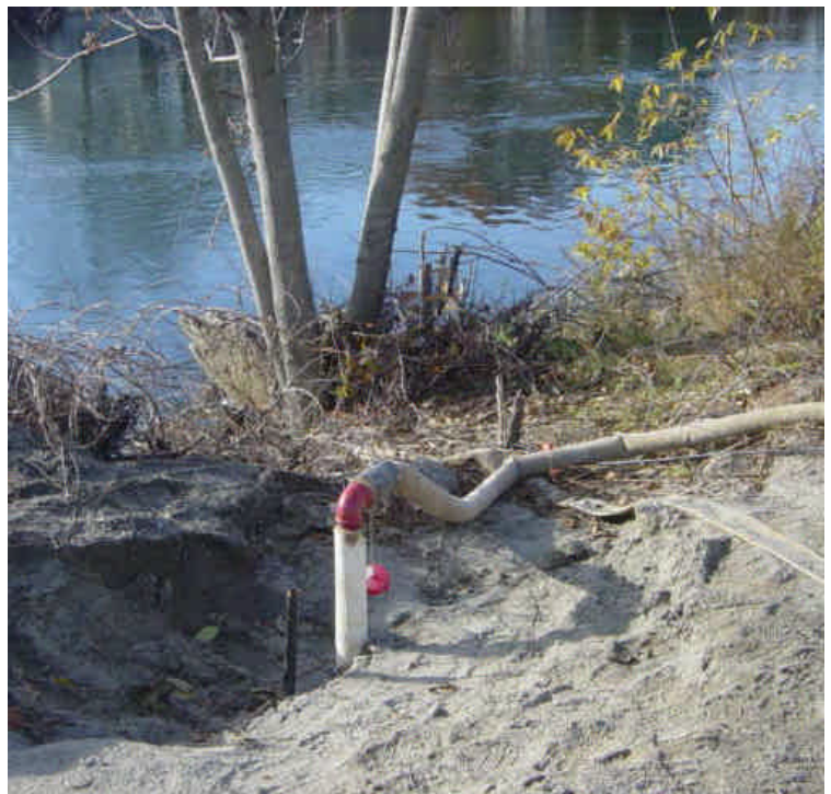
A water valve has been excavated on the northeast side of Ash Creek leaving an area of exposed soil adjacent to the bank. The exposed soil has the potential to run-off into the water.
