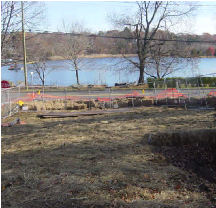
On the west side of the Saugatuck River, the previously exposed soil at the regraded drilling pit, has been stabilized with hay mulch.
