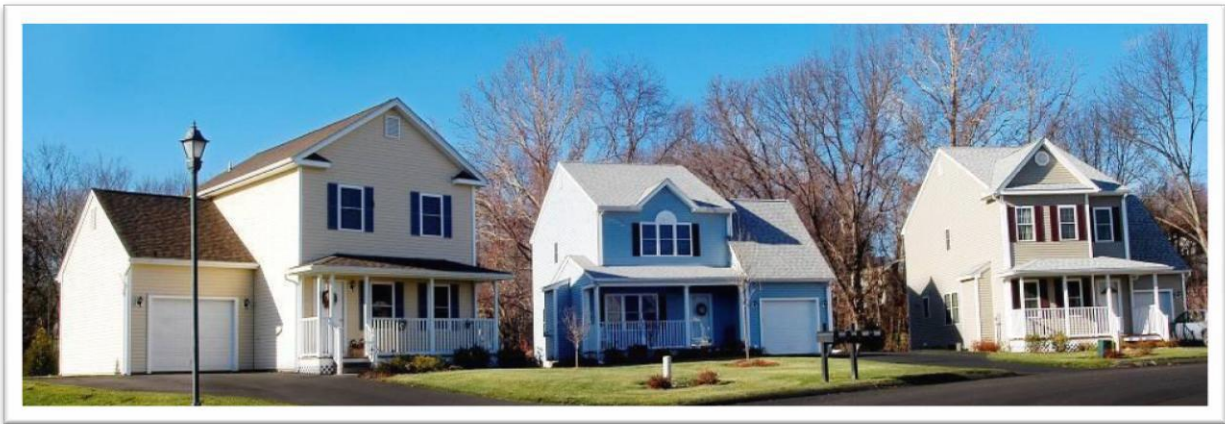
The Olde Oak Village in Wallingford incorporates attractive affordable and market rate homes. Photo Credit: Partnership for Strong Communities
