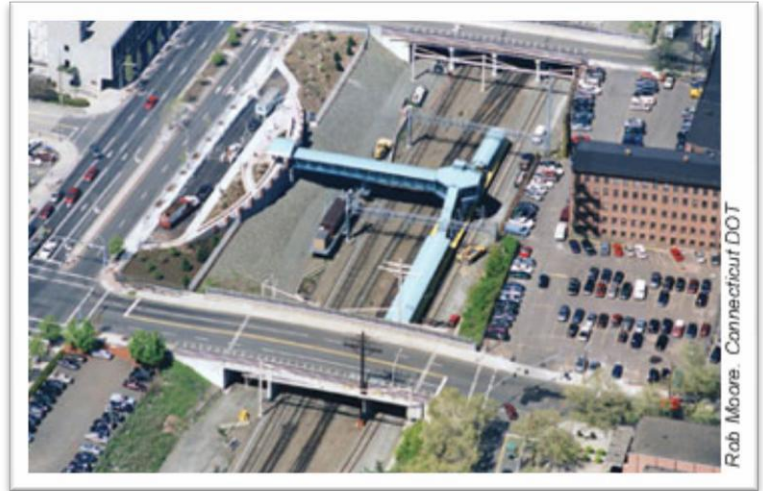
Aerial view of the new State St. Station in New Haven
