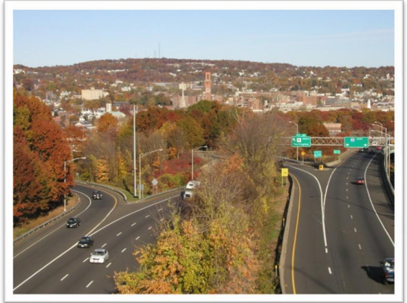
Approaching the I-84/Route 8 Interchange known as the "Waterbury Mixmaster" Photo Credit: Joe Perrelli, COGCNV
