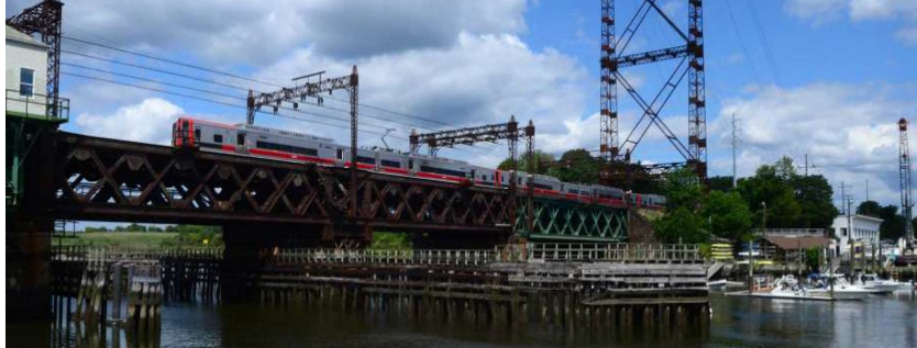
Figure 7: Walk Movable Bridge
