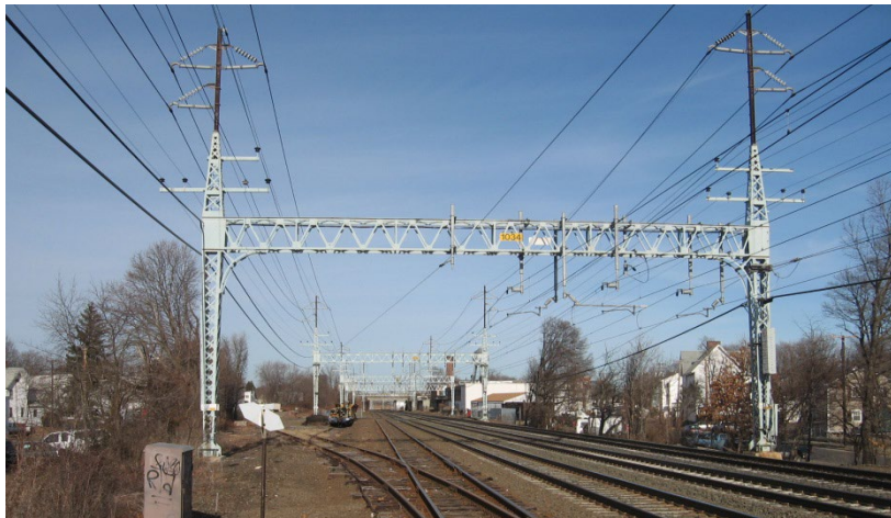
Figure 8: Catenary Structures on the New Haven Main Line
