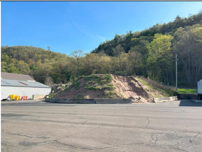
Ring sand pile with hay bales. Concrete blocks are used on site, as seen above.
