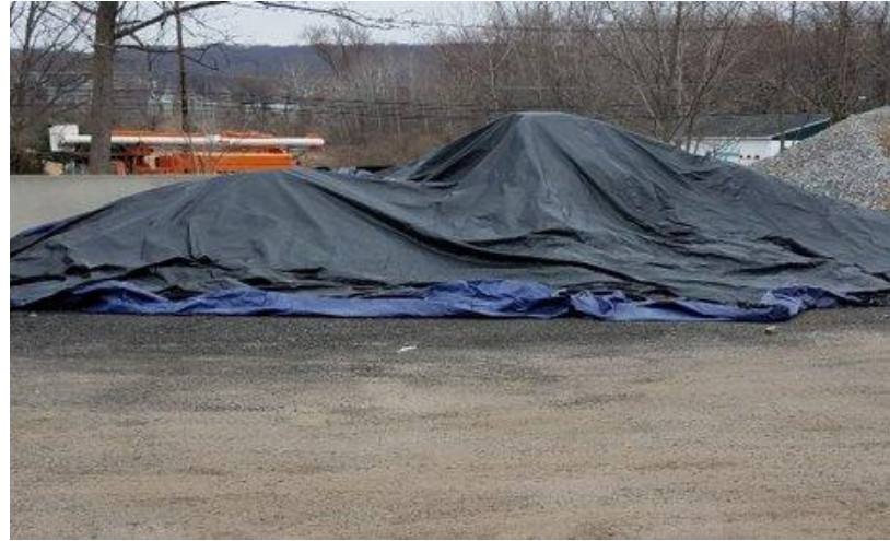
Cover piles of stored material to the extent possible. See example above.
