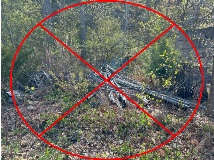
Elevate and cover galvanized steel with tarps to the extent possible.
