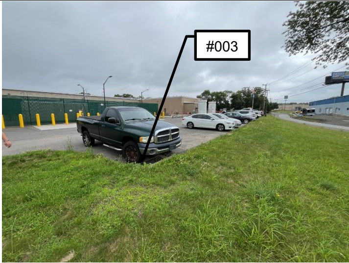
Outfall #003 located on the east of the Site. Outlet pipe within the catch basin structure is Outfall #003.
