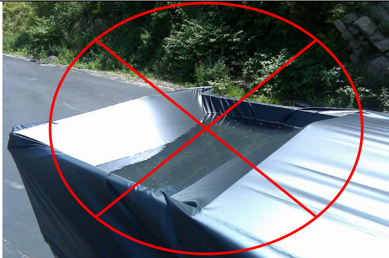
All dumpsters should have covers and drain plugs intact.
