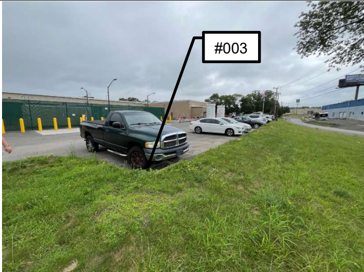
Outfall #003 located on the east of the Site. Outlet pipe within the catch basin structure is Outfall #003.
