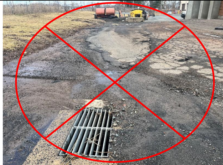
Maintain pavement and sweep loose material around catch basins.
