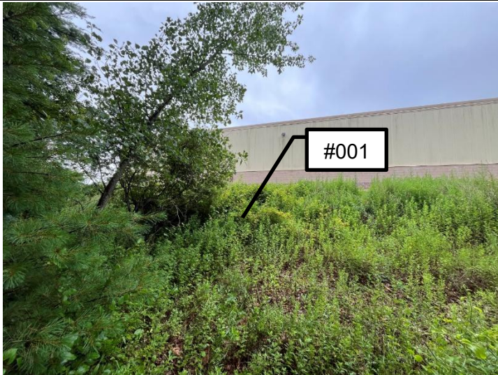
Outfall #001 located on the west of the Site. 15" RCP at the toe of the slope behind the Bridge Building.
