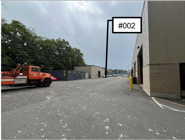
Outfall #002 located on the northeast of the Site. Outlet pipe within the catch basin structure is Outfall #002.
