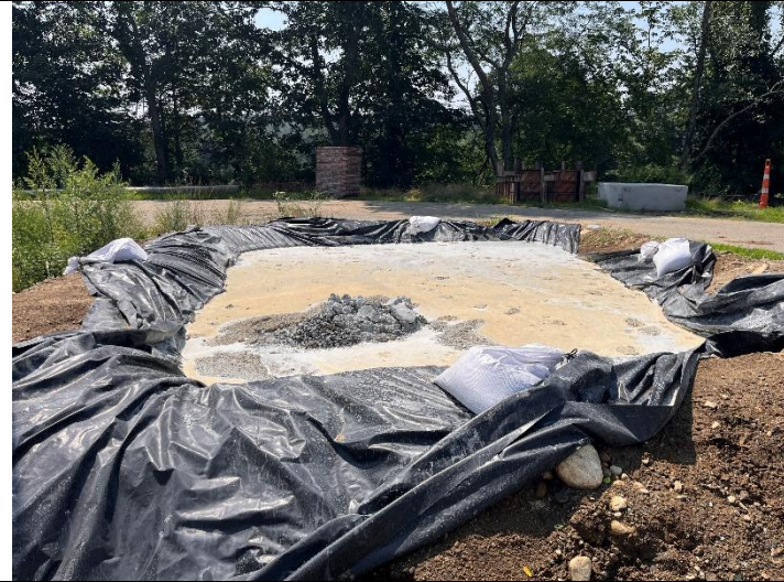
Concrete clean-out should be contained for proper disposal.
