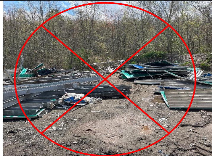
Cover piles of stored material to the extent possible.
