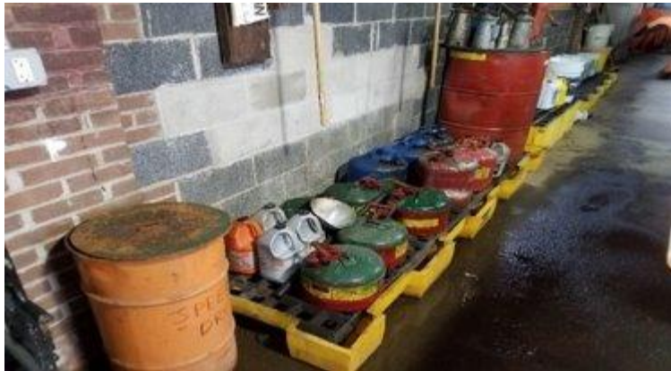
Label and contain hazardous chemicals. Keep spill containment and chemicals free from stormwater and stormwater run on.
