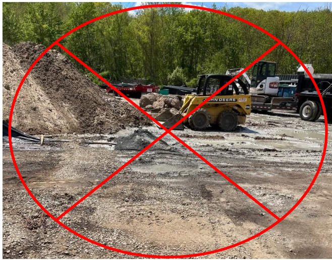
Concrete clean-out should be contained for proper disposal.
