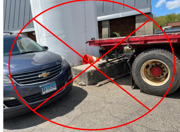
Keep area around magnesium chloride tank free from parked vehicles and stored material to the extent possible.
