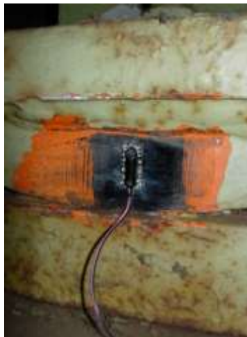
Figure 27: An installed foil strain gage on the Meriden Bridge
