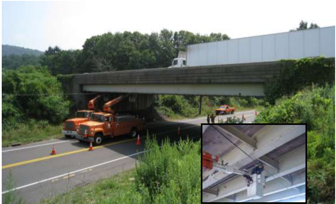
Figure 1: Installation of the dual BHM/BWIM system on the Meriden Bridge.
