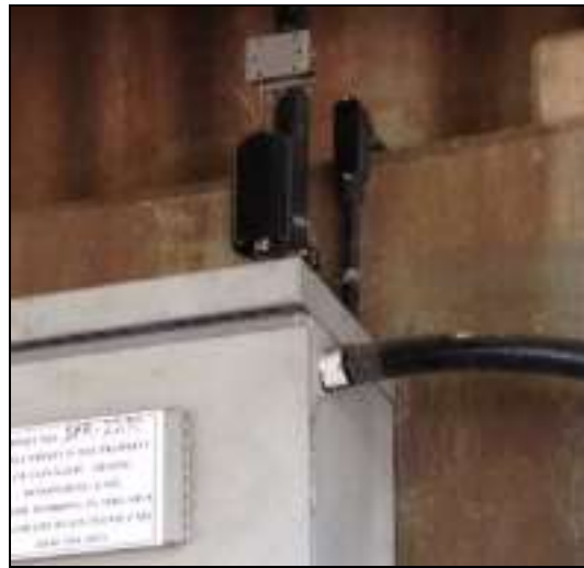
Figure 14: Microphone to measure global vibration of bridge
