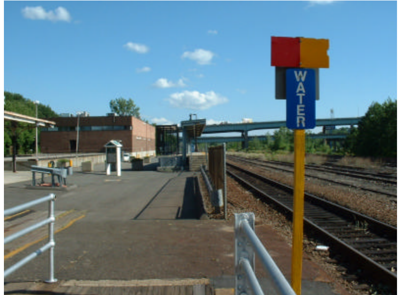
Replace Fence, remove highway guide rail, return fencing to building fence, provide gate
