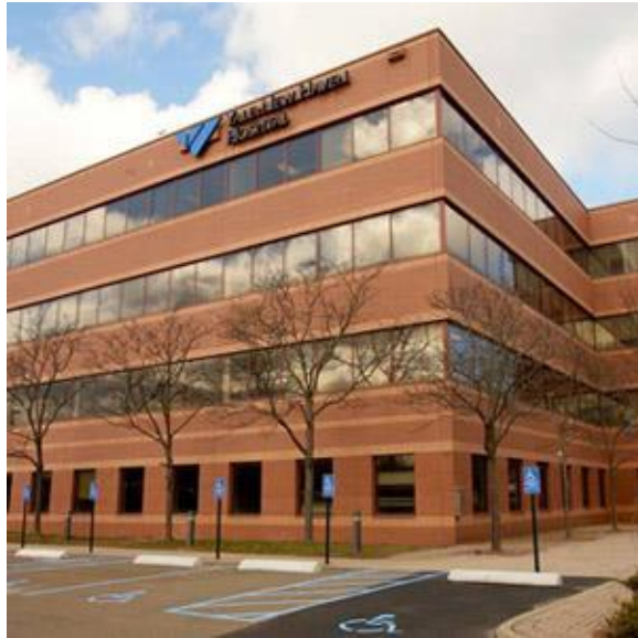
NORTH HAVEN MEDICAL CENTER (PHOTO CREDIT: YNH)
