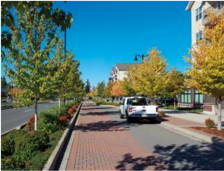
Permeable interlocking paver installation at Joint Military Base Lewis-McChord (JBLM) in Washington State. Source: https://www.estormwater.com/bmps/military-base-installs-permeable-pavers-main-street
