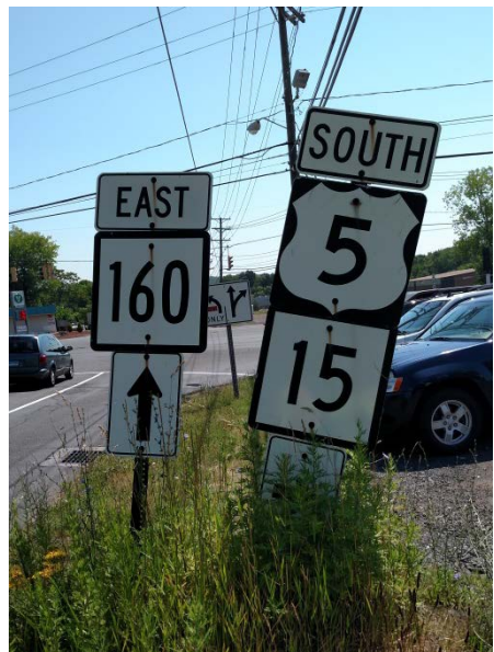
Figure 13. Signs Blocked by Overgrown Vegetation
