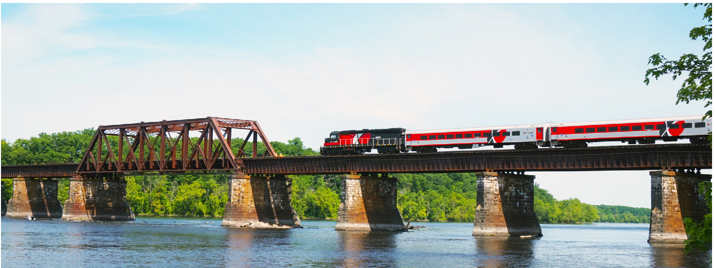
Figure ES-9: Hartford Line Train crossing the Connecticut River in Windsor Locks
