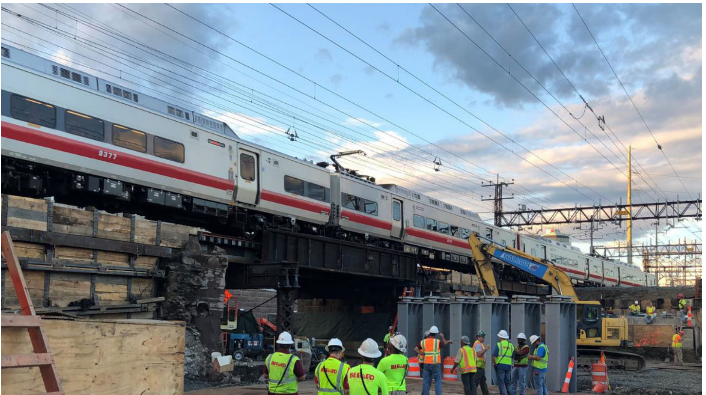
Figure ES-7: Stamford Construction Site
