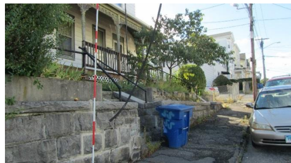
Figure 10: Hanging Overhead Wire on South Street
