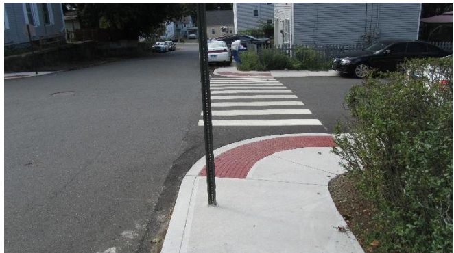
Figure 21: New Handicap Ramps at Lounsbury Street/ Fairmount Street
