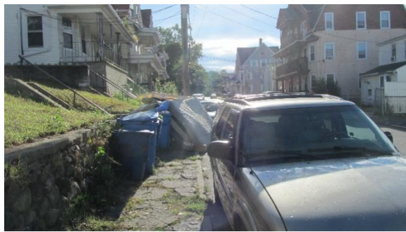
Figure 9: Trash Bins and Mattress Obstructions on South Street
