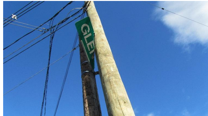
Figure 15: Glen Street Sign Bent between Two Poles
