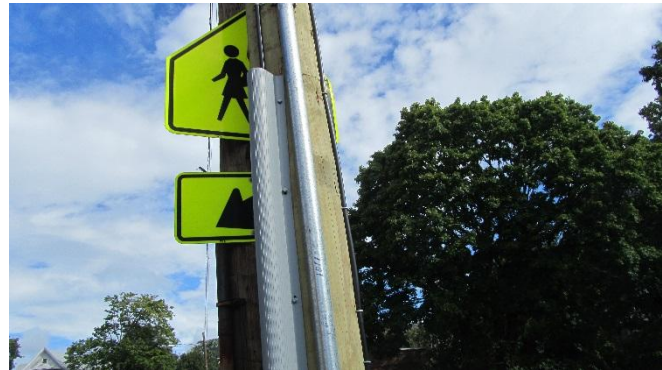
Figure 20: School Crossing sign hidden behind pole
