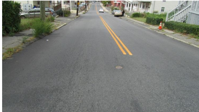
Figure 18: New Pavement Markings Along Washington Street
