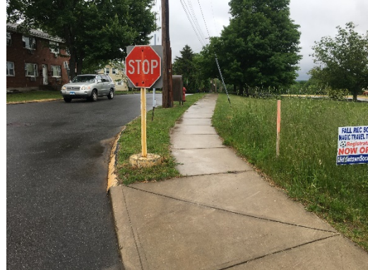
Figure 15: Sidewalk Along Maynard Street
