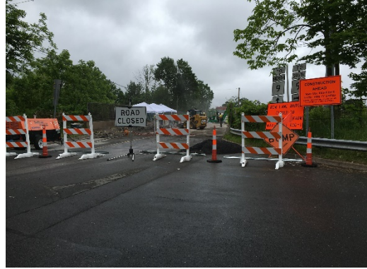
Figure 22: Construction at Top of Bow Lane
