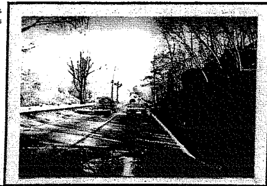
Spatial Enclosure from Woods and Rock Cut, SB past James Farm Road Bridge
