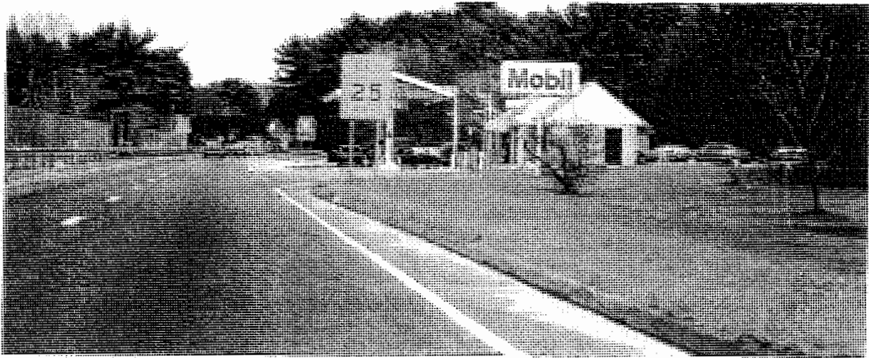
STATION 149+600 FAIRFIELD SERVICE AREA EASTBOUND, LOOKING EAST
