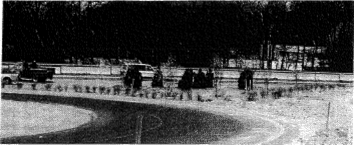
STATION 154-700 EXIT 47 OFF RAMP, LOOKING NORTH ACROSS MERRITT PARKWAY
