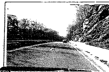
SB2 Topography/Rock Cut Exposed at Exit 29 (SB)
