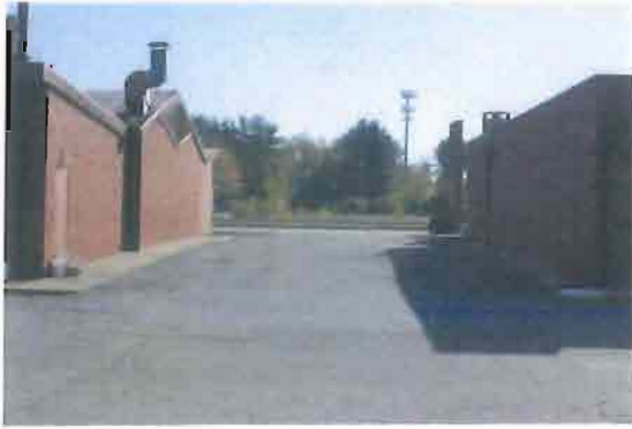
Photo #5: Roadway between both buildings, dispensary left building.
