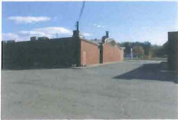
Photo #6: West corner of building overview.
