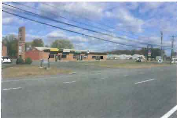
Photo #3: South corner front overview of building.
