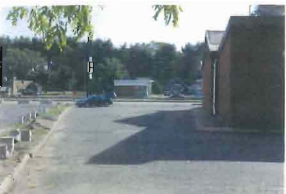
Photo #8: North corner of building overview.
