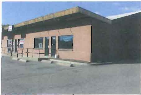
Photo #10: Overview east corner of building front entrance
