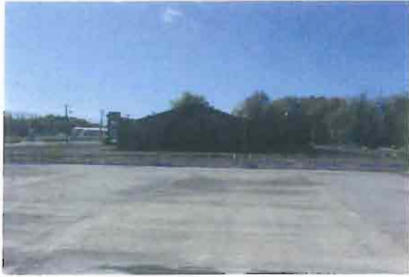
Photo #9: Northeast side building overview
