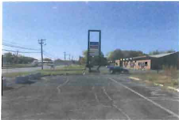
Photo #2: Front view looking towards south direction, east corner of building.
