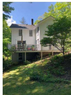
East Elevation of the House
