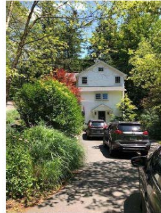
West Elevation of the House/Future Location of 2-Car Attached Garage
