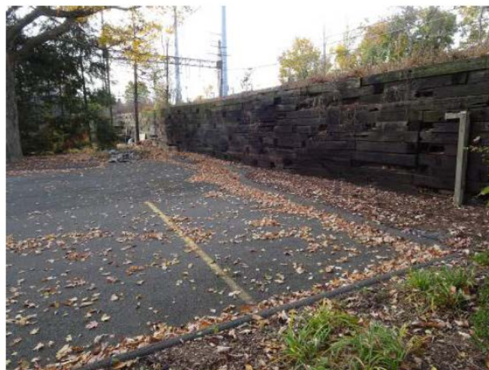
Wood retaining wall along Metro North rail line north end of Lot 10 to be rebuilt
