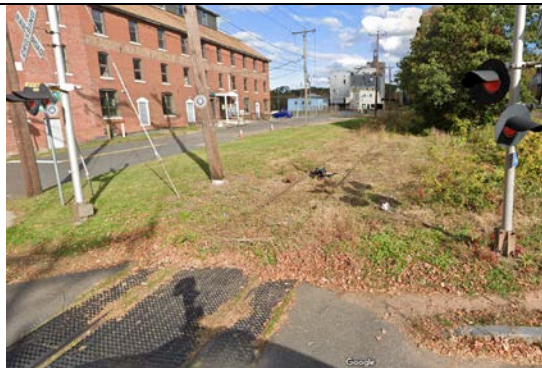
Oakland St intersection (courtesy: Google 10/2021)
