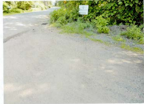
Buried railroad track at Mitchell Street looking east
