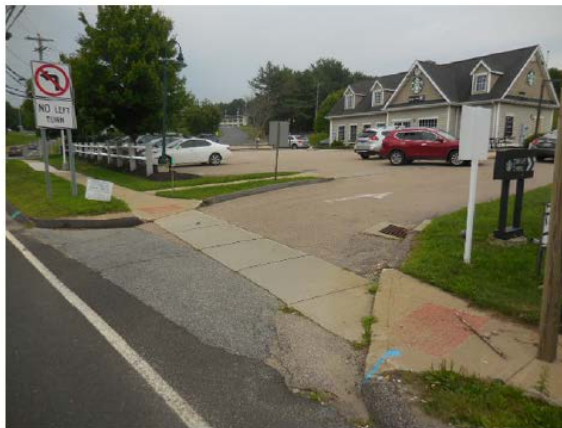
View facing northeasterly from Flanders Rd showing the acquired rights area
